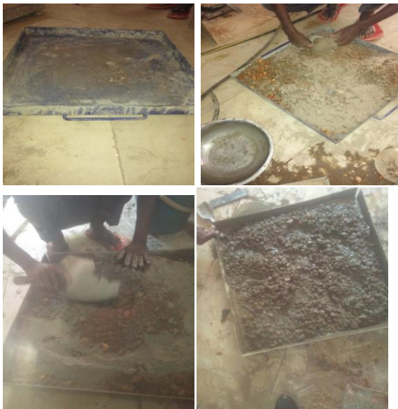
Figure 5: Preparing and mixing the concrete components
