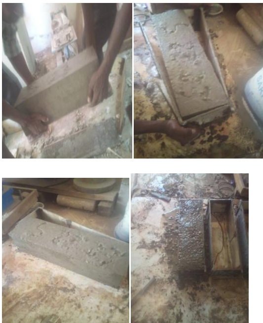
Figure 6: Manufacturing concrete beams
